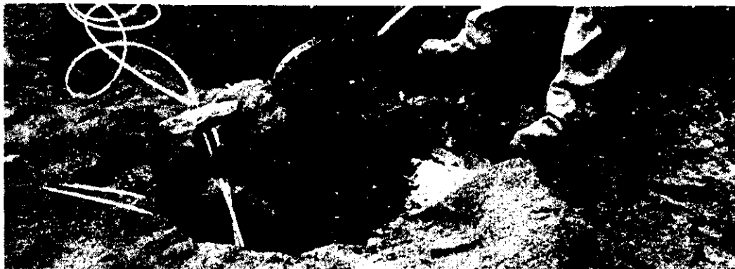
Figure 18. Proper stemming effectively reduces airblast.
