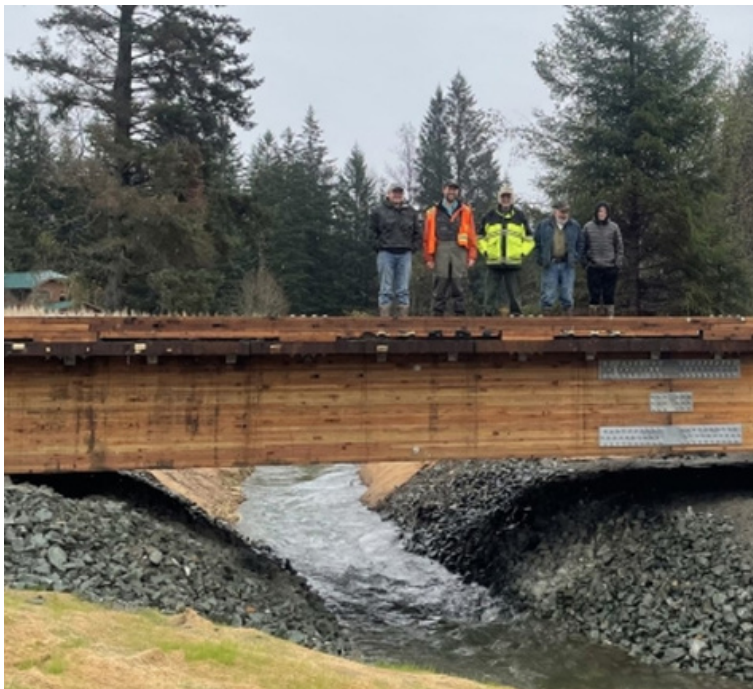
The new bridge as of October 2022.
