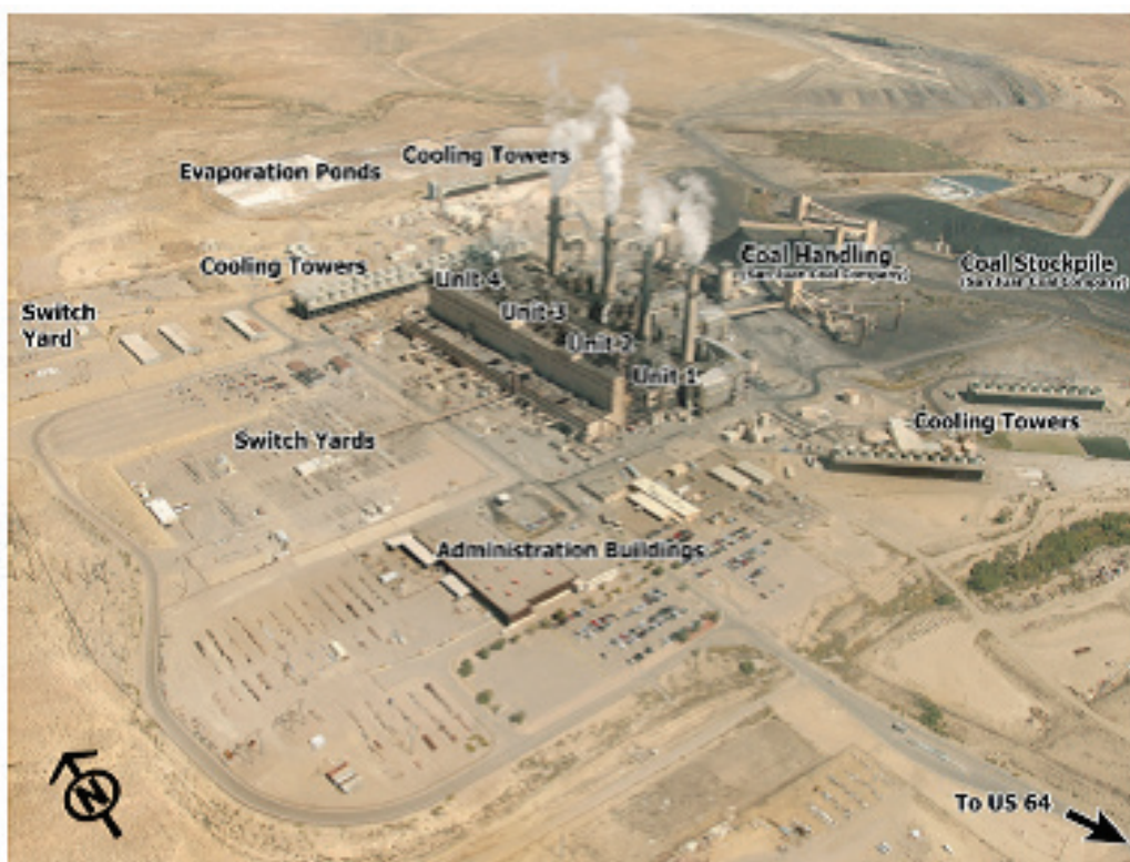
Figure 2.1-8: Overview of San Juan Generating Station Facilities
