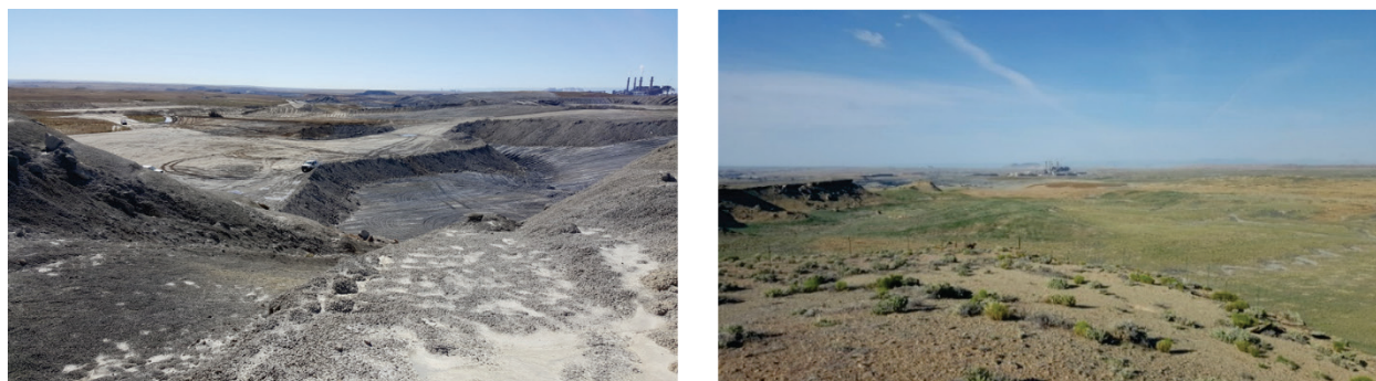
Figure 2.1-7: Photograph of Reclamation Activity and Completed Reclamation at Piñon Pit
