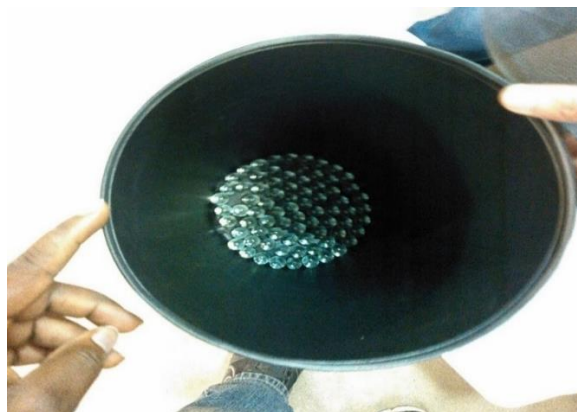
Figure T2.8 Glass marbles at the base of the column during construction
