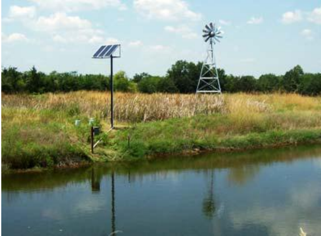
Figure 1 - Solar and wind re-aeration devices installed at the Rock Island No. 7 passive treatment system.
