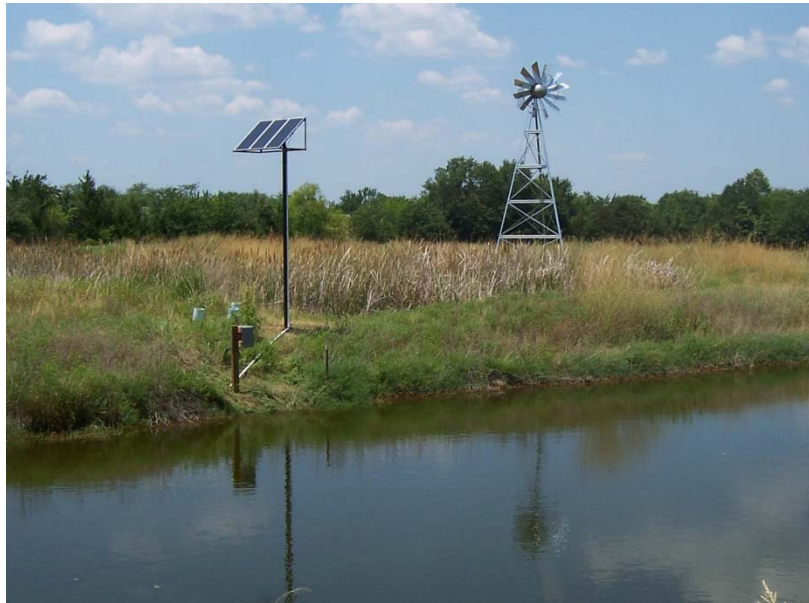
Figure 4.27. Solar panel (left) and windmill (right) placed on high terrace between Cell 1 (background) and Cell 3 (foreground).
