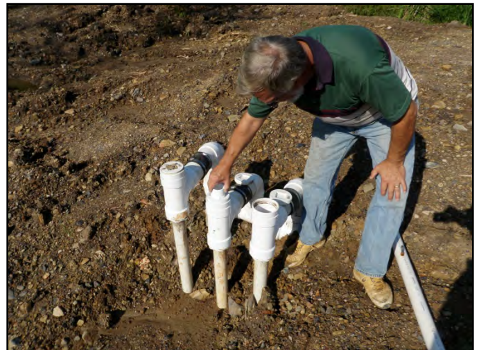
Trompe 1 was installed first (top) with Trompes 2 and 3 added later. Trompes 1, 2, and 3 are installed in series in order to generate compressed air, each trompe requires about 4 ft of drop from inlet to outlet (middle). Bruce Leavitt and BioMost, Inc. personnel installing Trompes 2 and 3 (middle). Dye testing (bottom left) illustrates improved dispersal of AMD in an aerated pond (bottom left). Inspection of Trompe 1 air inducers (bottom right).
