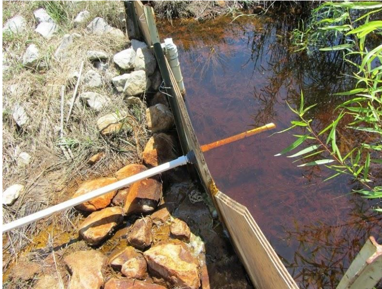
Figure 5: Photograph of weir constructed along with installed PVC to channel AMD into the test cells. A continuously-recording flow sensor is installed in the adjacent PVC stilling well.
