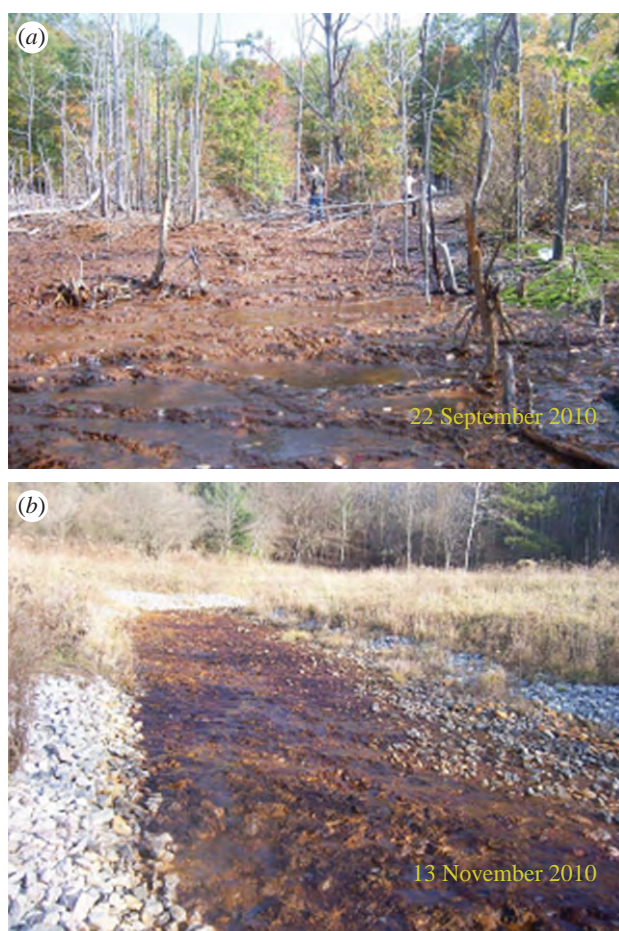
Figure 4. A natural iron oxide mound at Brubaker Run, Cambria County, PA (a), and an engineered 'oxidation/precipitation channel' at Dents Run, Elk County, PA (b). In both systems, the accumulation of Fe(III) minerals is due to low-pH Fe(II) oxidation by micro-organisms. (Online version in colour.)
