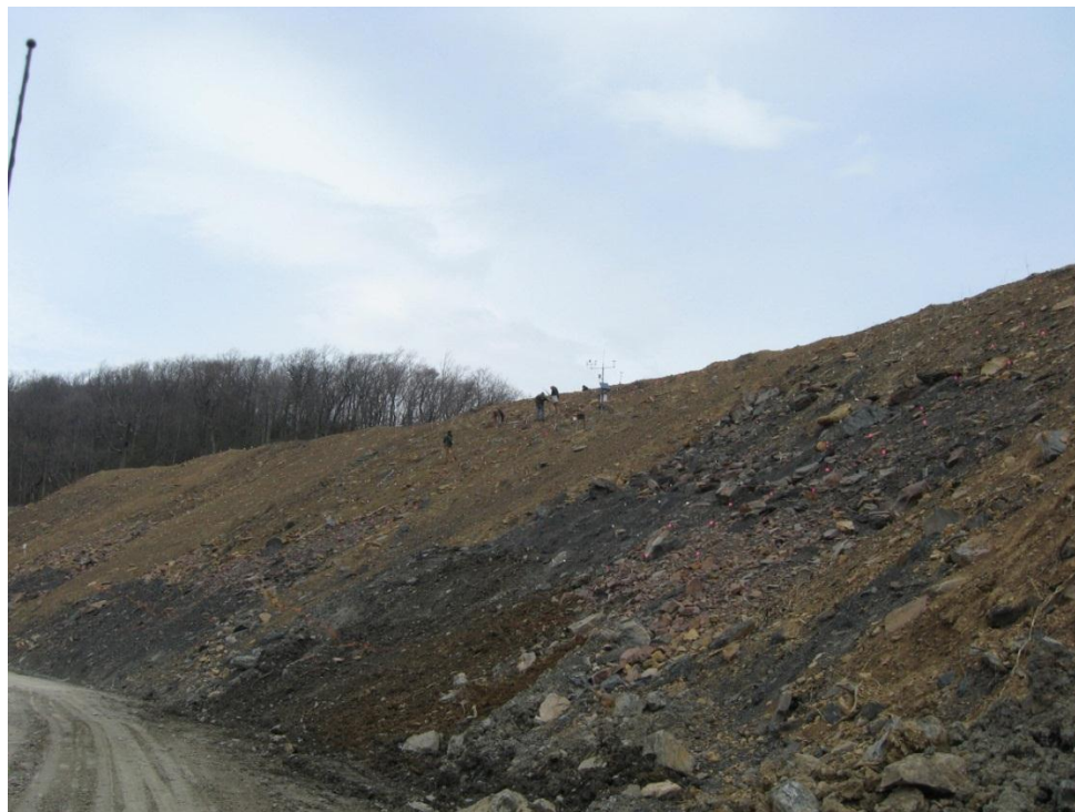
Figure 2-5 Premium site after the FRA reclamation process and during the installation of the weather station.
