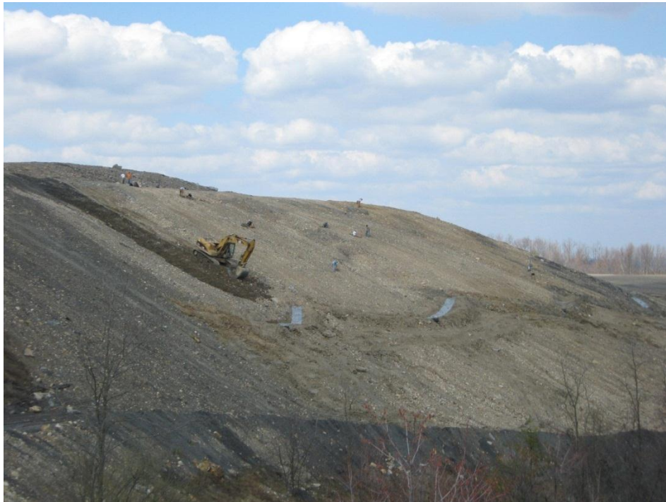
Figure 2-4 National site after the FRA reclamation process and during the construction of earthen berms. The tan sandstone surface layer can be seen in the surface materials to the right of the track hoe.
