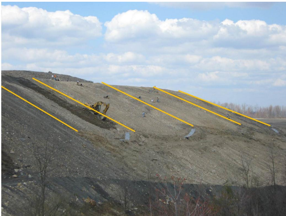
Figure 2-7 National site subdivided in plots by earthen berms (yellow lines).
