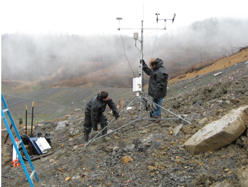
Figure 2-9 Installation of the weather station at Mountainside site.
