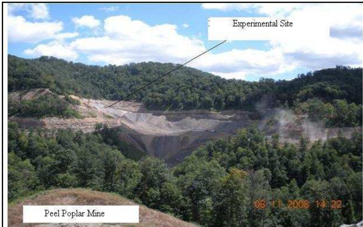
Figure 3.12: Experimental site at the Peel Poplar Mine (before highwall elimination)
