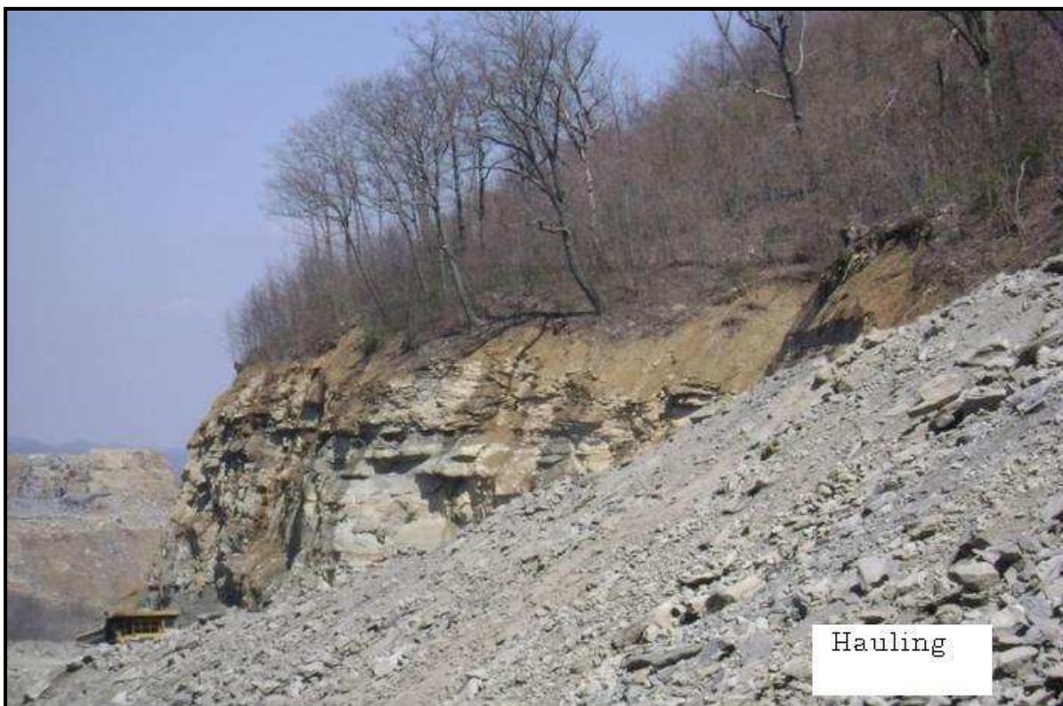
Figure 3.14: Hauling of spoil material
