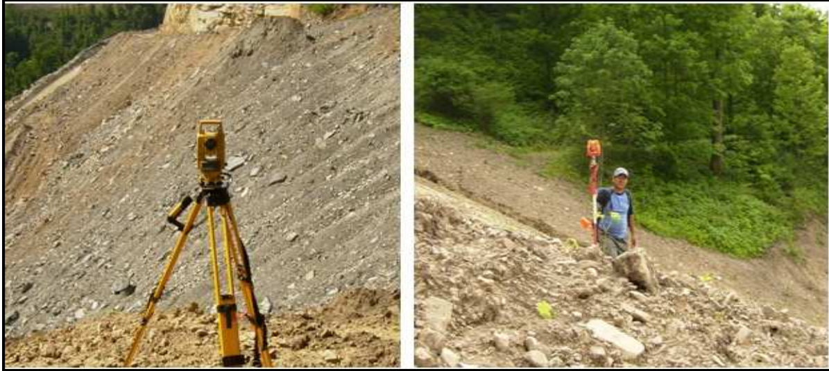
Figure 3.18: Combination of total station and prism for survey work
