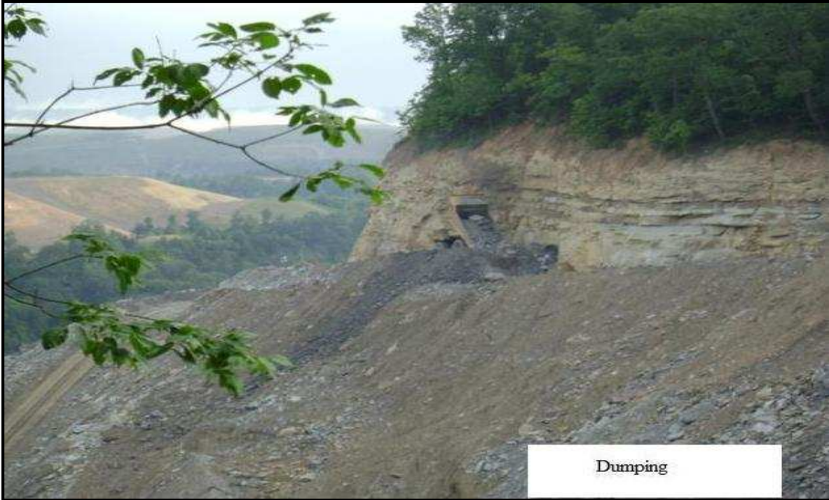
Figure 3.15: Dumping of spoil material
