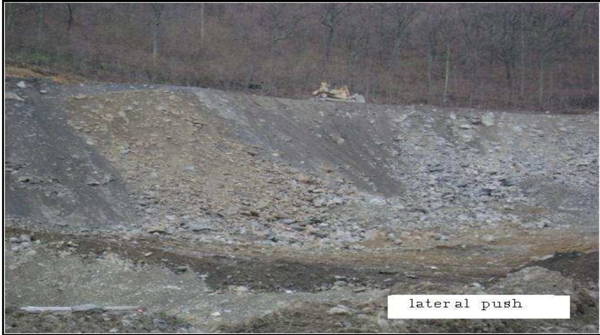
Figure 3.16: Lateral pushing of spoil material
