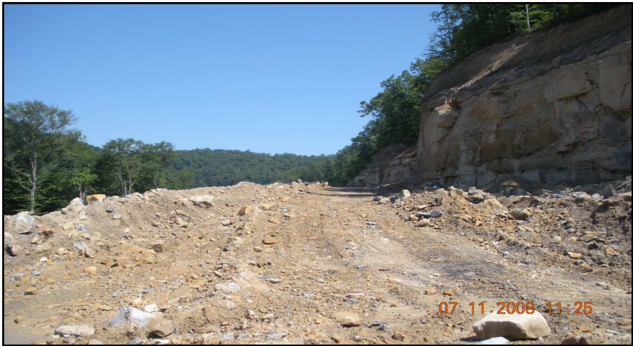
Figure 3.2: Contour haulback with horizontal lifts
