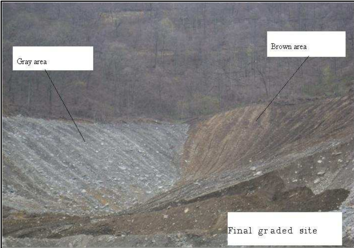
Figure 3.17: Experimental site after final grading
