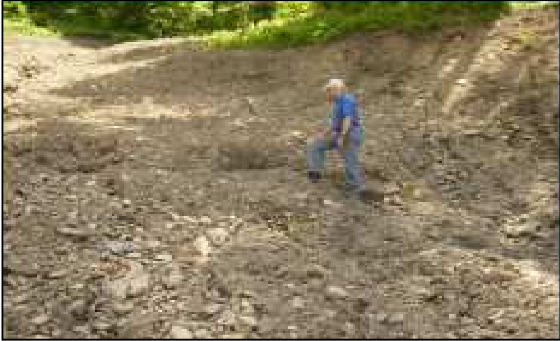
Figure 4.4: Small slumping in the brown spoil area after two heavy rains
