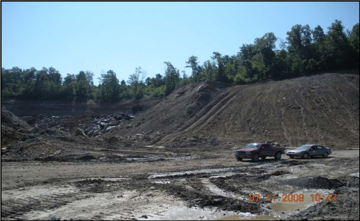
Figure 3.6: Final graded highwall (North and South Surface Mine Logan County, WV)
