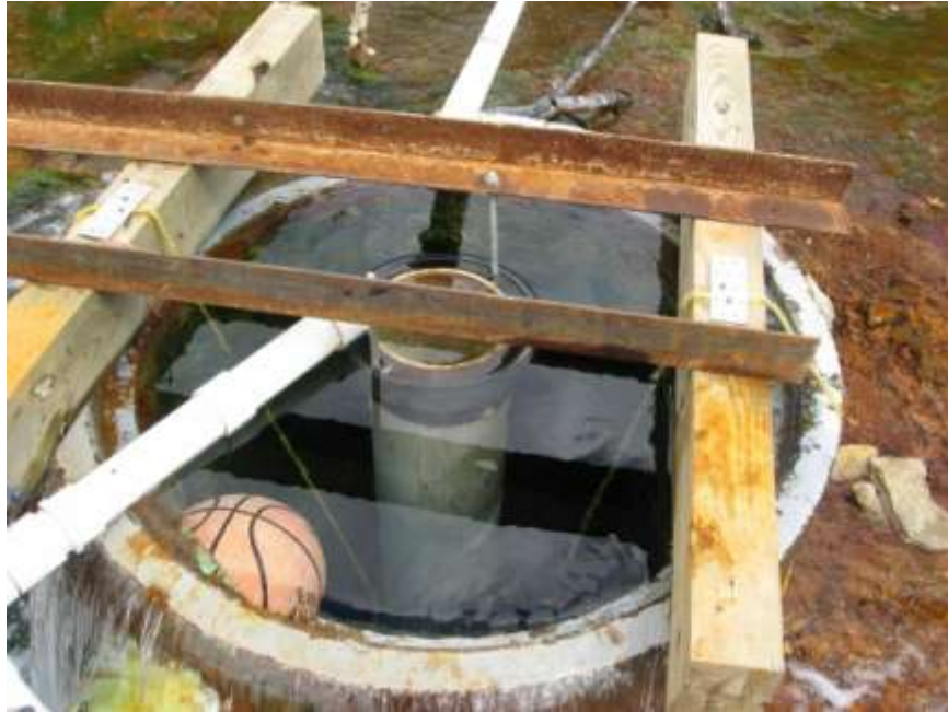
Figure 20. Eight inch pipe adjusted to water surface with sampling pipe in position.
