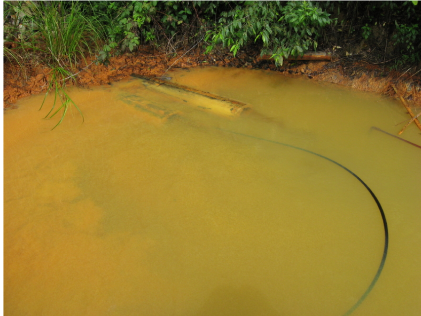
Photo 20. T&T #2 Discharge pipe with sampling pipe inserted.
