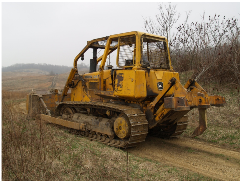
Figure 2. D-6 grade bulldozer with 32-inch ripper attachment used to rip soil at field site.
