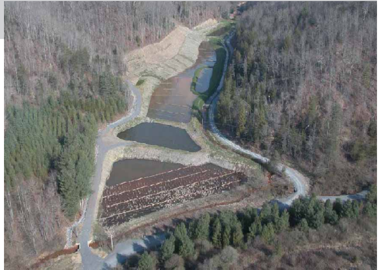
ABOVE PHOTO: Aerial photograph of SAPS implemented in Ely Creek.
