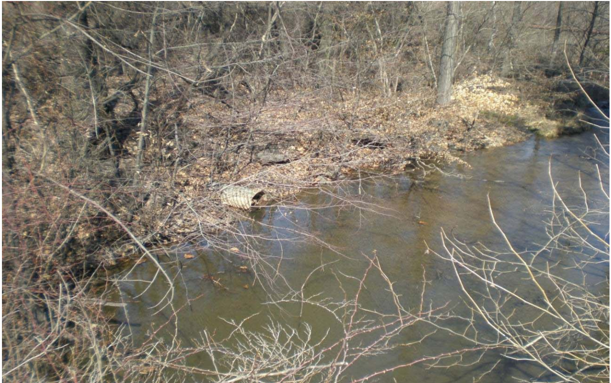
Fig. 19. View looking from road at LBC-5 at culvert pipe.
