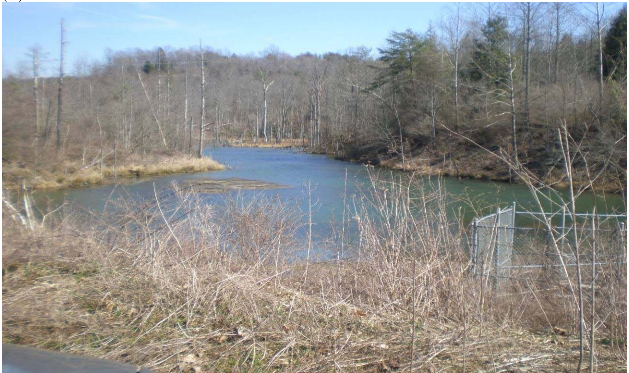
Fig. 10. (A) Downstream view of LBC-1 toward LBC-3 and (B) upstream toward LBC-1 from end of pond just before LBC-3.
