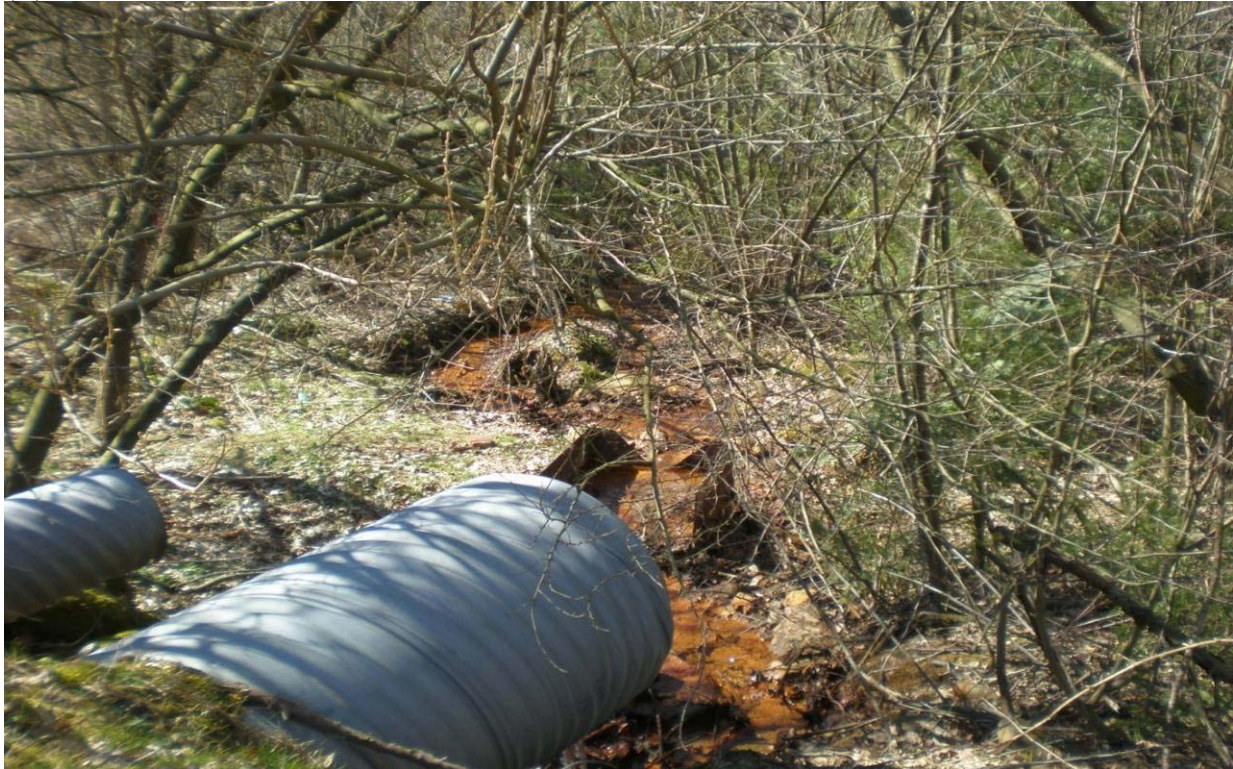
Fig. 4. (A) UD-2 seep origin and (B) UD-2 discharge with weir.
