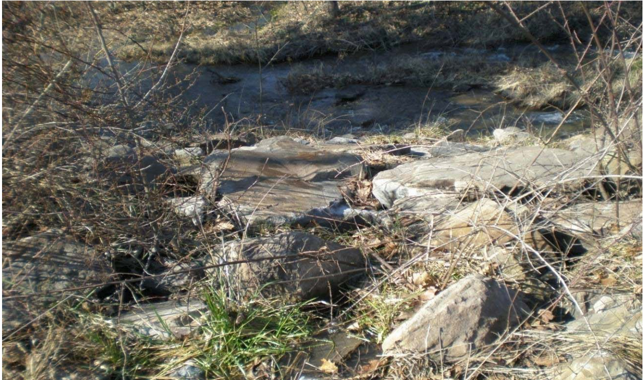
Fig. 23. View from LD-5a discharge to creek just above LBC-5.
