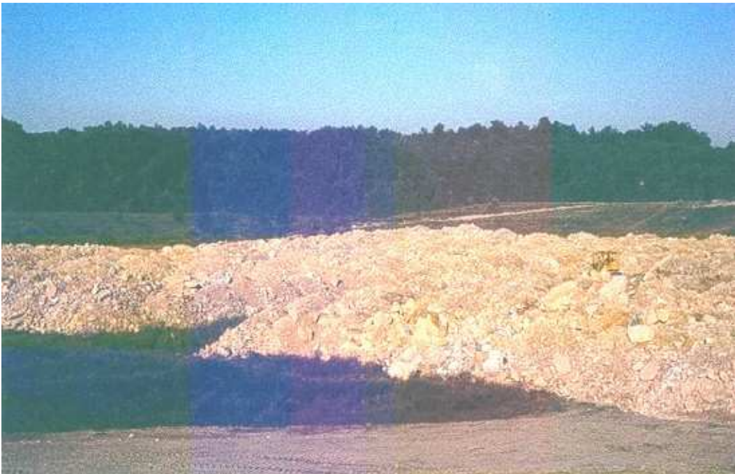
Figure 4.2.3 A newly constructed loose-dumped reclamation plot at the Starfire Mine planted in 1996. (Conrad, 2002)
