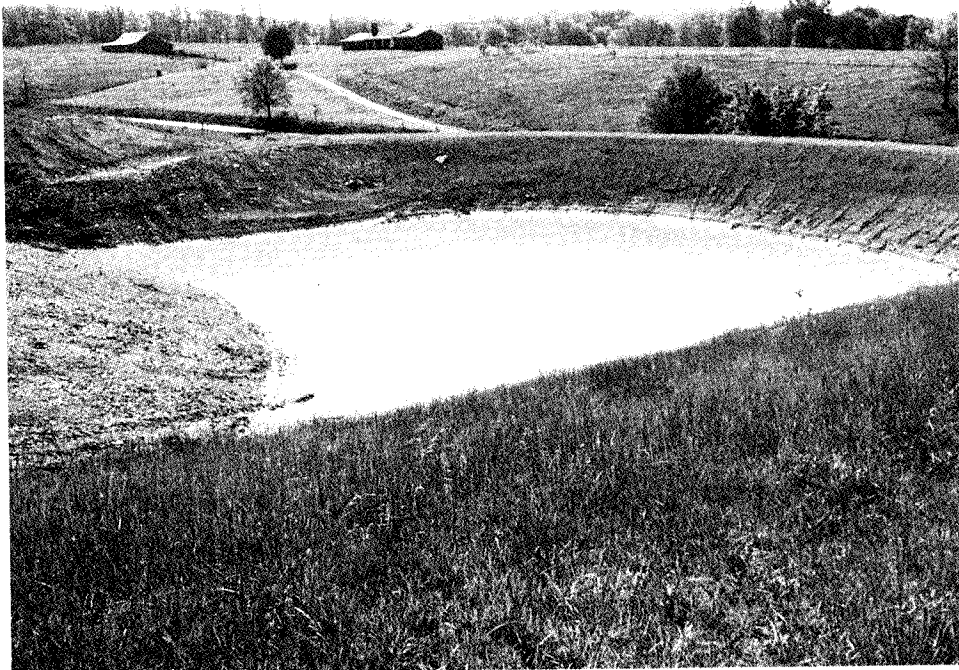
Sedimentation ponds are constructed prior to mining to prevent off-site stream damage.
