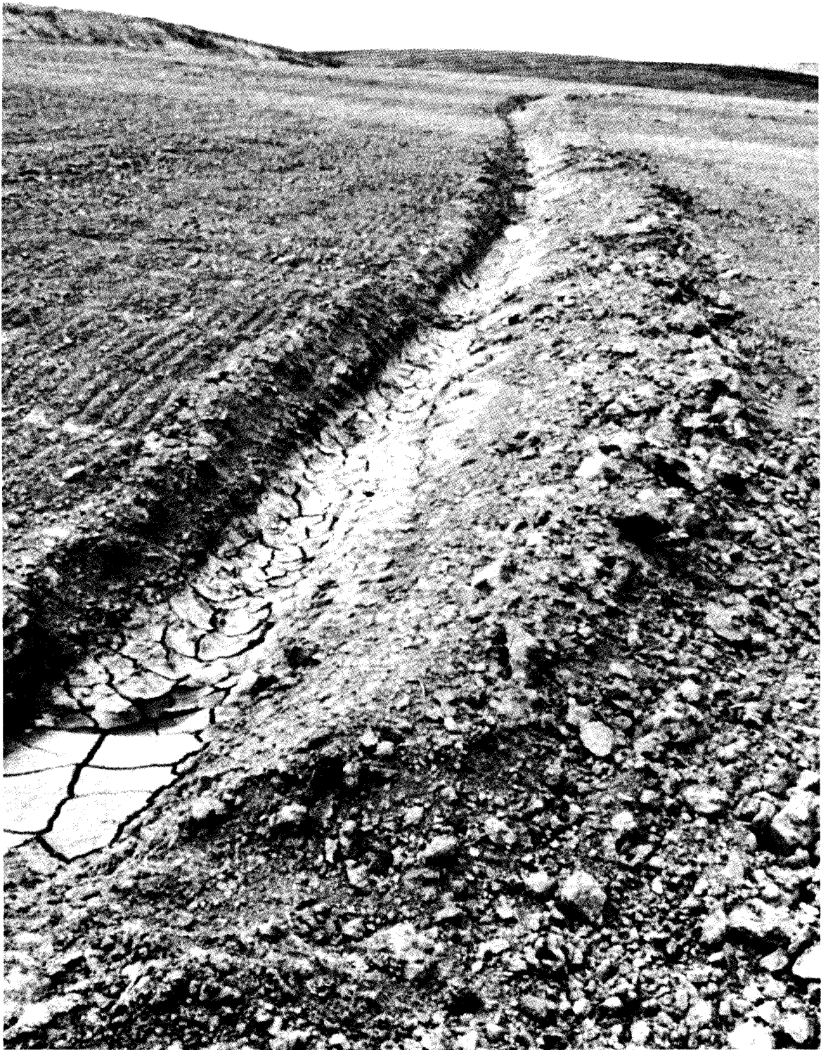
Energy dissipating diversion ditches are used to minimize erosion by breaking up long, smoothly graded slopes.
