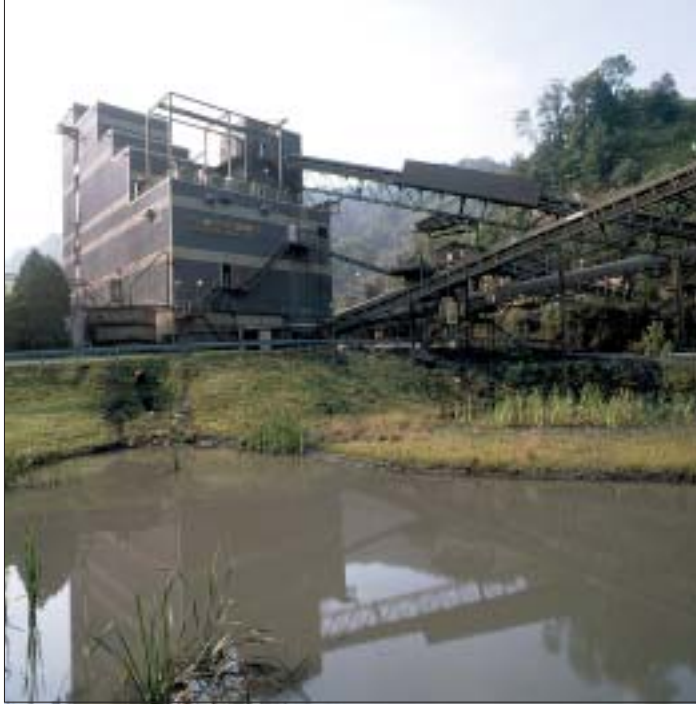
Coal preparation facilities are used to prepare coal for market. Coal is brought from the pit to the preparation plant where it is separated from rock or overburden, washed, and sized for shipment. Under the Surface Mining Law preparation facilities are permitted and regulated just as the mining operations. And, when the operation is completed, the preparation facilities must be removed and the land reclaimed.
