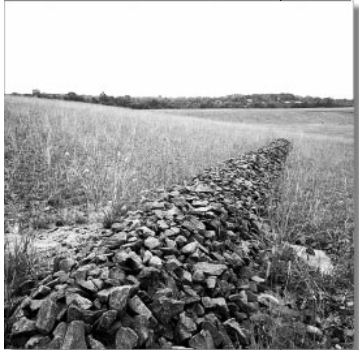
In areas of high rainfall conditions water can easily erode soils. To prevent erosion of the hillside at this Pennsylvania mine site, a rock check dam was constructed across the slope. This small structure slows the flow and prevents water from eroding gullies in the smoothly graded slopes.
