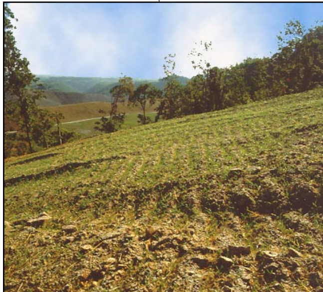
Bulldozer tracks across the slope provide niches that trap runoff for use by grass seedlings.
