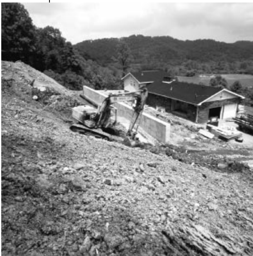
A landslide above this Kentucky house required emergency work to prevent further damage. Surface and subsurface drains at the top of the hill divert water around the house. The concrete wall will provide a solid base at the bottom of the hill and prevent future sliding. The large pipe covered with gravel behind the wall will prevent water build-up and keep added pressure off the wall. As the last step in the abandoned mine reclamation process, the entire site will be graded and revegetated.
