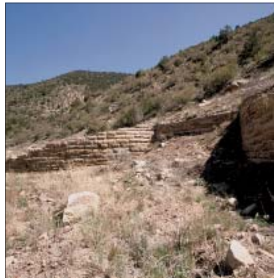
At this Utah site, abandoned portals and open mine shafts were closed to eliminate dangerous conditions. During reclamation the portals were backfilled and the larger portals that were flanked with historic Italian-cut sandstone retaining walls were closed; but, preserved the historic stone intact. Today, with reclamation complete, these structures are an historical feature and a reminder of the Italian miners of the early 1900's who built houses, walls, and other structures using rock from the surrounding canyons.
