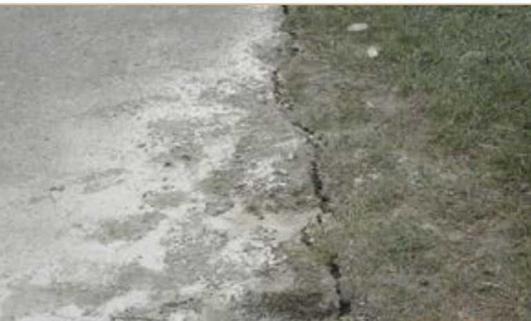
The crack that appeared while contractors were injecting concrete into the shaft areas.
