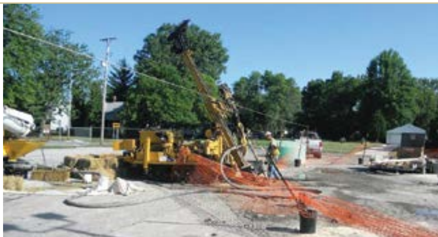
Contractors begin grouting the holes to ensure proper stabilization of an abandoned coal mine shaft near Jerome Elementary School.
