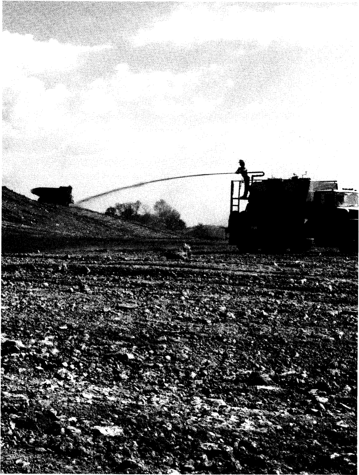
Planting with a hydroseeder.
