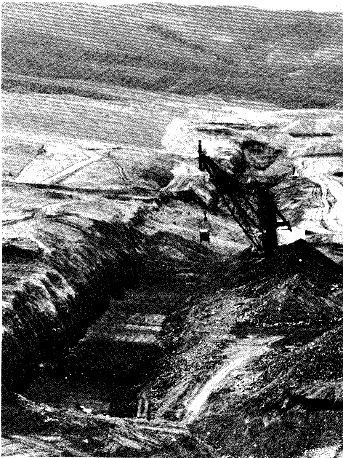
Dragline removing overburden at area type mining operation.
