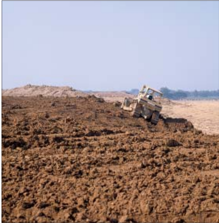
Topsoil removal and handling are especially critical in the Midwest where prime farmland must be restored to its former productivity level. After the final grading of spoil, the topsoil at this site was hauled to the reclamation area and is being spread evenly over the land by bulldozers. This mining company replaced all the soil to prime farmland depths (48 inches), even though much of the acreage was classified non-prime farmland where soil could have been replaced at the 12-inch depth required for non-prime farmland. However, the operator's commitment to extra soil replacement has restored the land to a level capable of supporting a wide variety of current and future agricultural uses.
