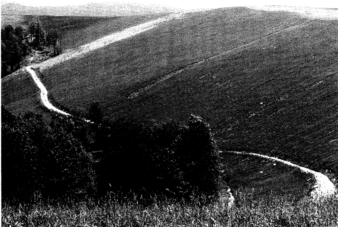
Reclaimed contour surface mine to approximate original contour.
