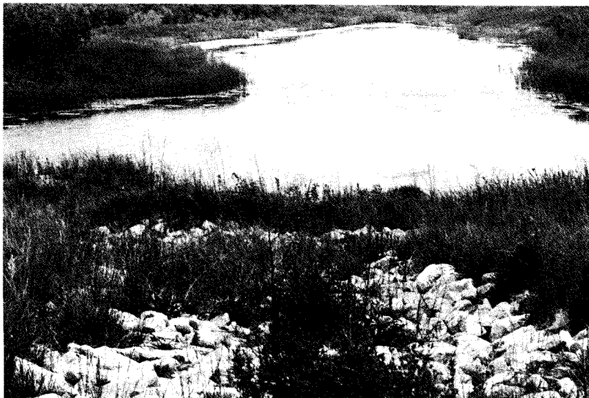
The construction phase of this experimental practice, to create a wetland wildlife habitat, involved direct planting of a slurry pond without covering it with four feet of clean material.
