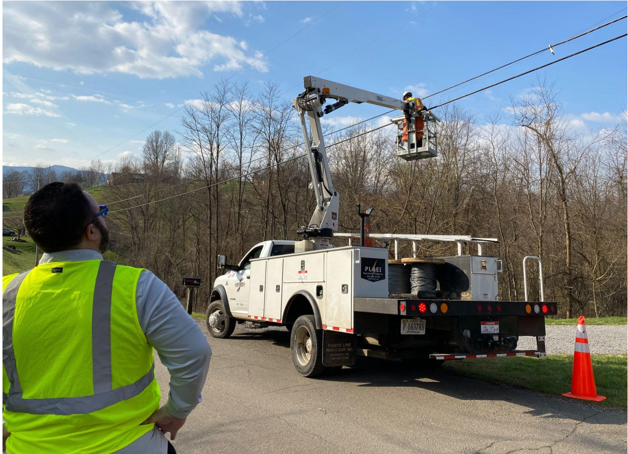
Point Broadband installs new fiber optic cable in Lebanon, VA.
