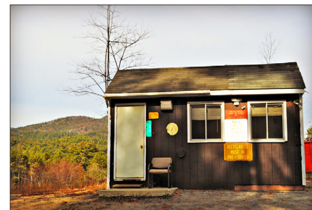
A small attendant building provides a comfortable work space and has a small room, tool storage, and restroom.
