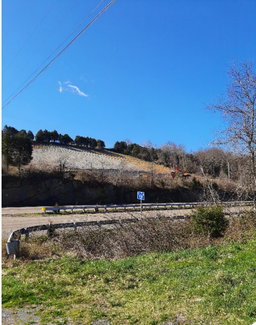
Jonah work continues on Rt. 19 access Rd.
