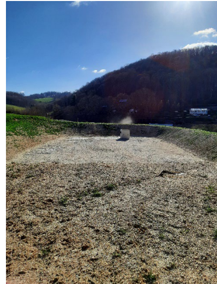
Jonah ,sediment basin on Tazewell County access rd.
