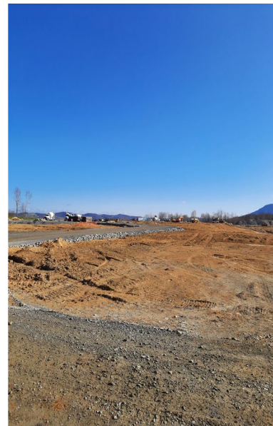
Jonah near building pad
