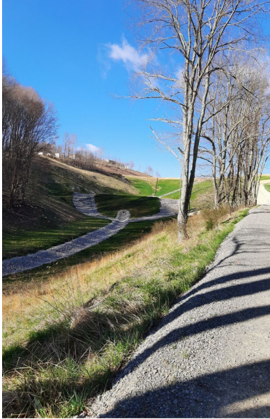
Jonah riprap channel from basin on Tazewell County line
