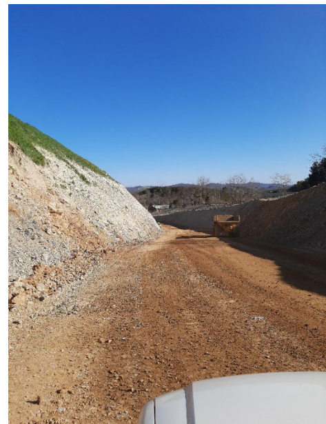
Jonah, work continues on Rt. 19 access road.
