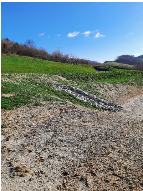
Jonah,sediment basin on Tazewell County access rd.
