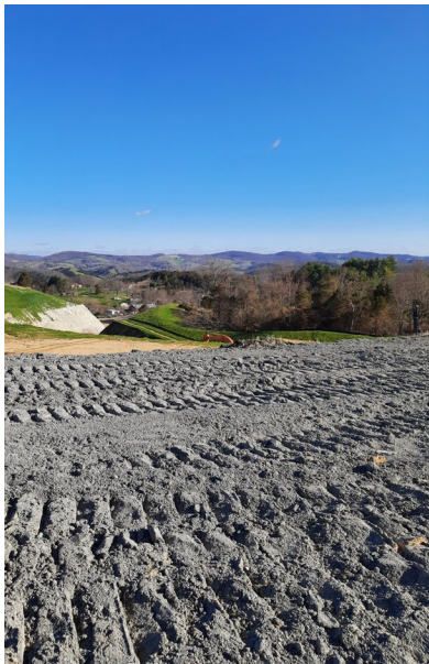
Jonah, Rt. 19 access road looking north
