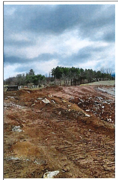
Rt. 19 Sediment Basin
