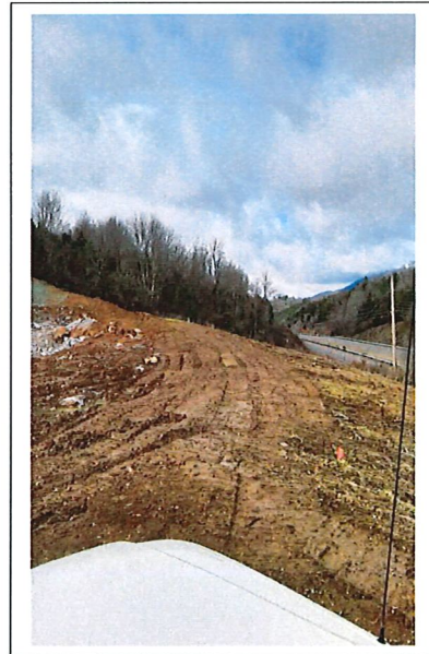
Rt. 19 Sediment Basin
