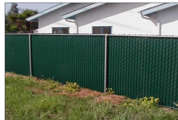
Chain link fencing is used with a green privacy fabric that enhances both security and aesthetic appearance of the transfer station.
