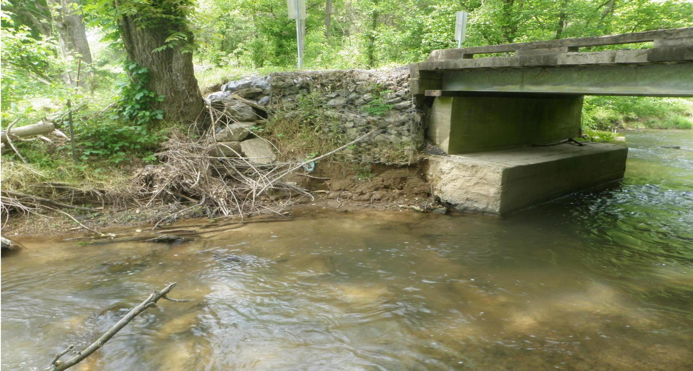
Area of new wingwall – downstream side Abutment B
