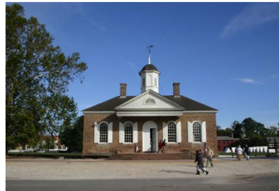
Historic Williamsburg Courthouse
