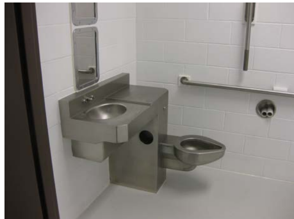
Isle of Wight Court Floor Holding Cell
