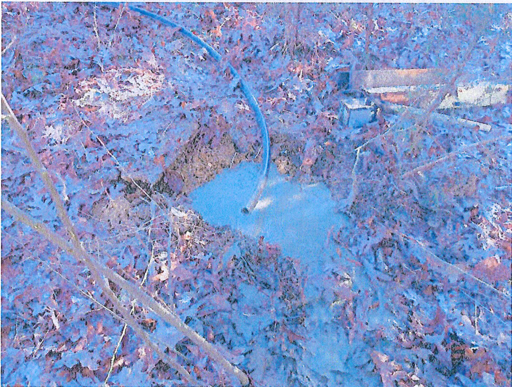
PHOTOGRAPH 6. View of gas boundary probe BP-1 with cement surface plug. Representative of abandonment procedures at all gas boundary probes.
