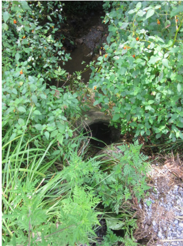
Photo 7: View 5' end-section at Culvert #2 that will be reinstalled. (8/8/18 by E. Virts)
