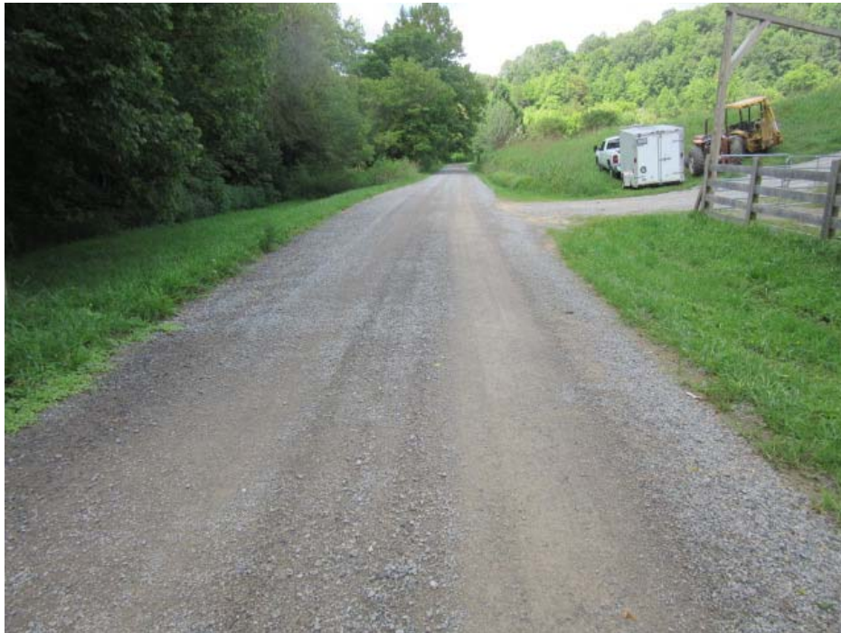
Photo 8: View of Rte. 678 at Culvert #2. (8/8/18 by M. Bolling)
