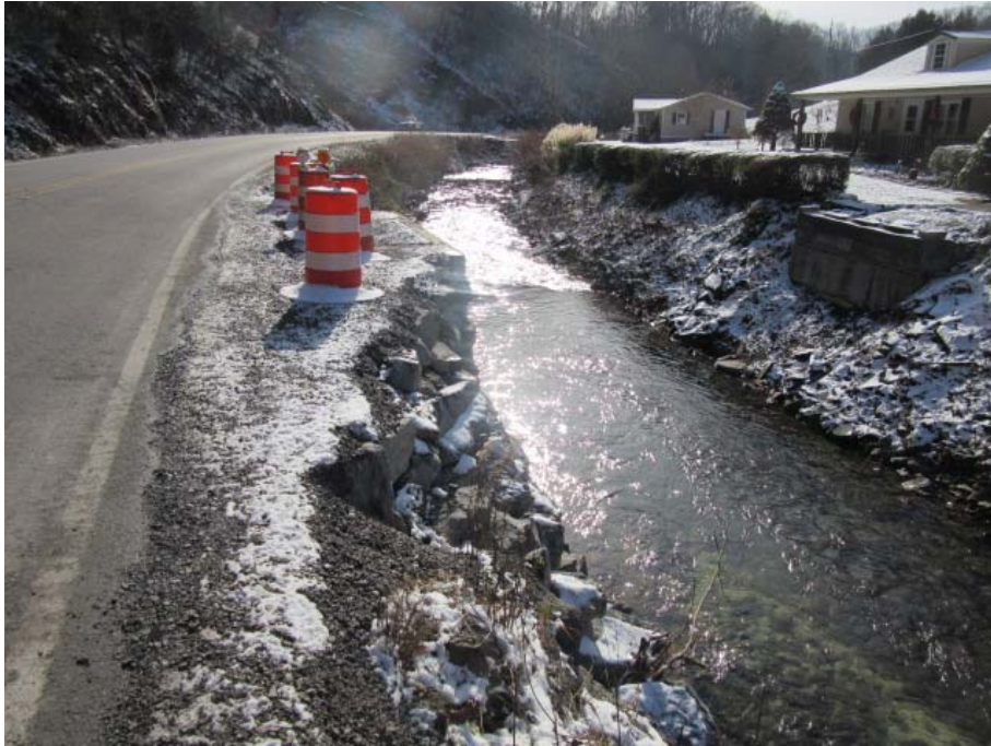
Photo 5: View looking south at stabilized stream bank/shoulder. (12/6/18 by M. Bolling)
