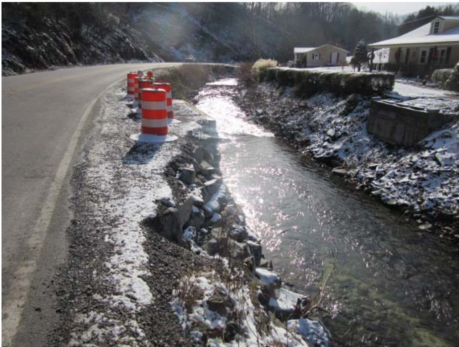
Photo 6: Another view looking south at stabilized stream bank/shoulder. (12/6/18 by M. Bolling)
