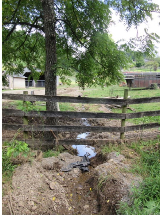
Photo 5: View looking upstream of Culvert #2. (8/8/18 by E. Virts)
