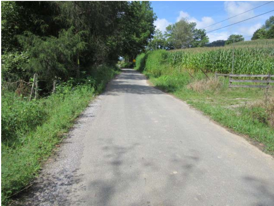
Photo 4: View of Rte. 678 at the location of Culvert #1. (8/8/18 by M. Bolling)
