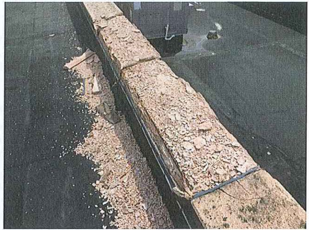
Disintegrating precast
