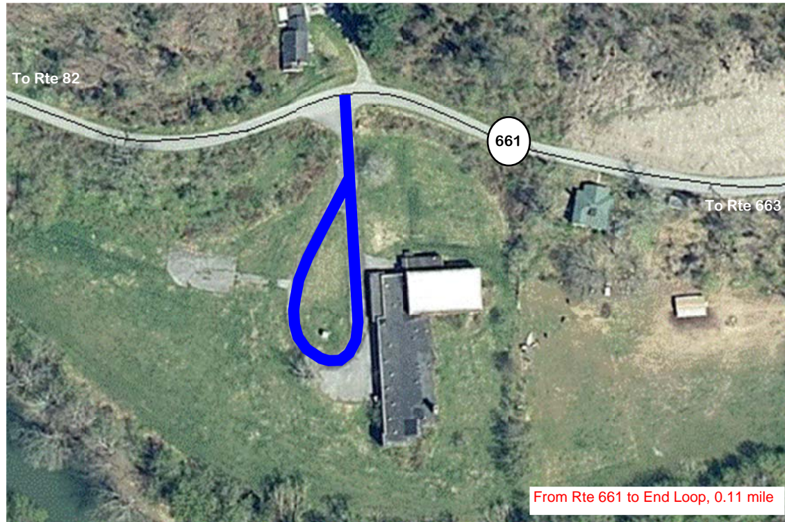
RTE 9532: CLEVELAND ELEMENTARY SCHOOL
