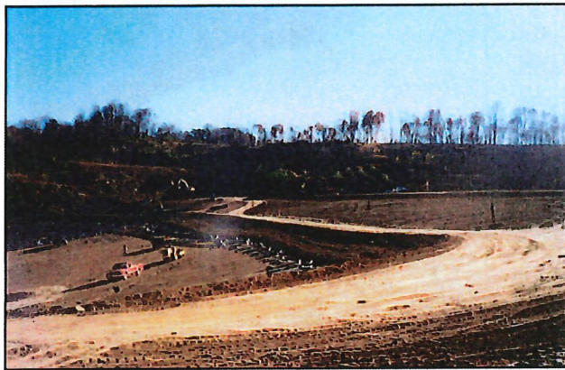
Construction of the cap system was completed in phases. A buttress was constructed over the face of the landfill to flatten slopes to 4 horizontal to 1 vertical to improve stability of the cap.
