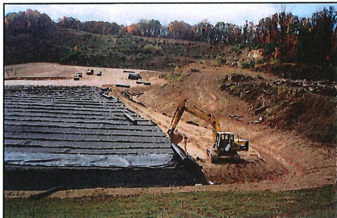
The project included construction of a 19-acre geosynthetic cap system.
