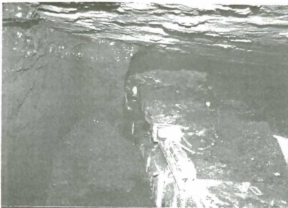
No. 2 Offset left side showing extent of last continuous mining machine advance in Drainway entry
