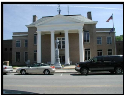
Tazewell County Courthouse
