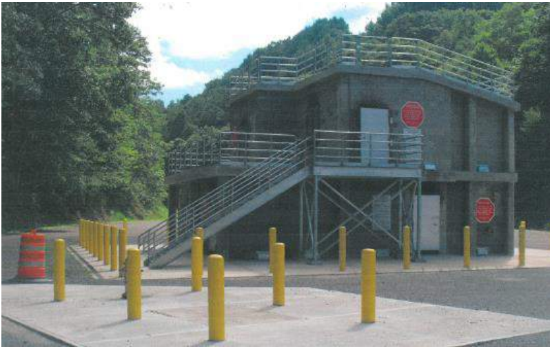
Richlands Fire & Rescue Department Burn Building
