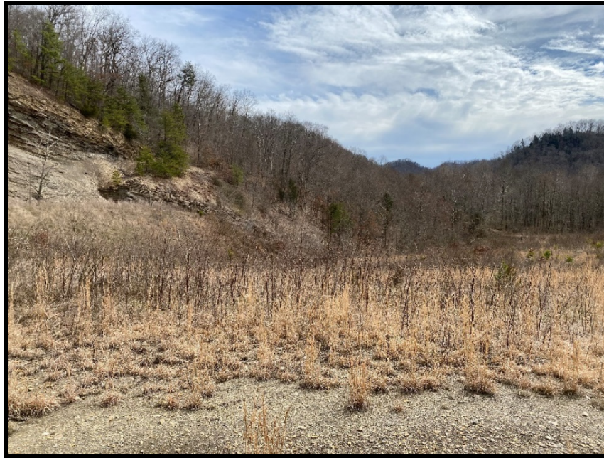
Figure 41: Kiser Pond Spillway – Northwestern Border of Property
