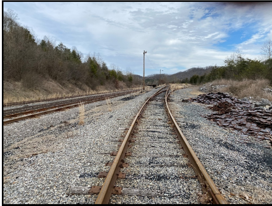
Figure 29: NS Railroad Tracks-Northern Boundary
