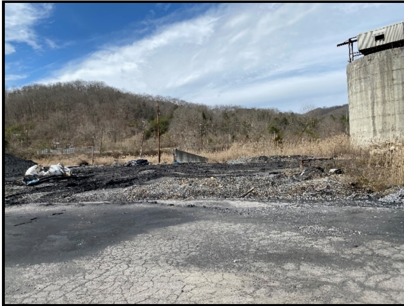
Figure 33: Reclaim Tunnel-Debris-Silo On Adjacent Property
