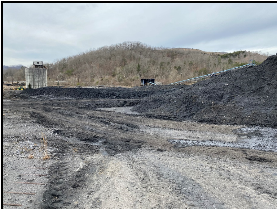
Figure 6: Northern Adjacent Property – Russell County Reclamation, LLC
