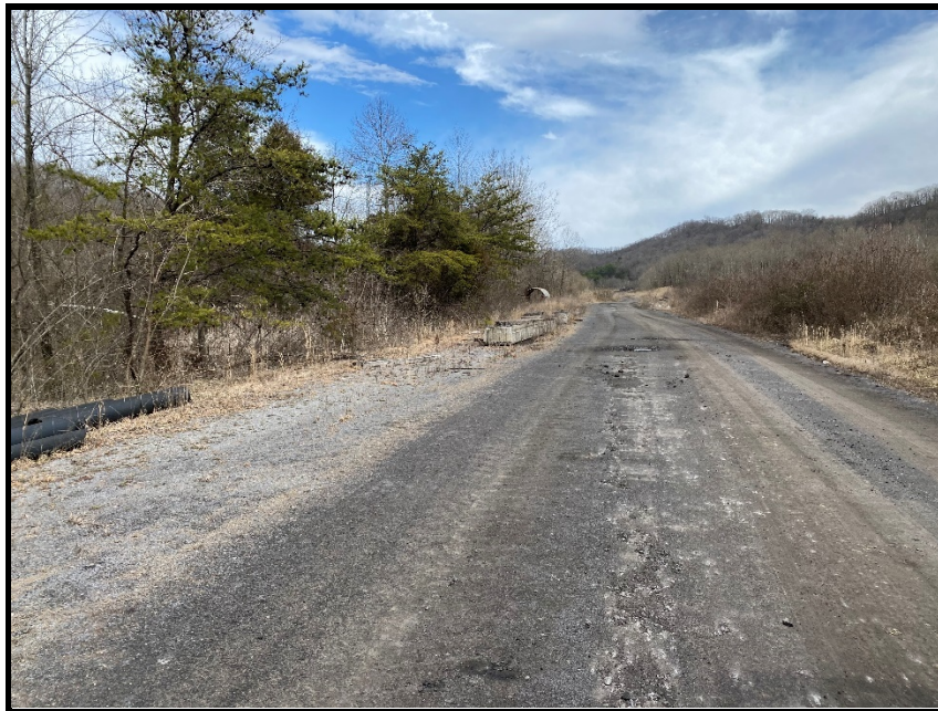
Figure 36: Access Road – General Debris (1 of 2)
