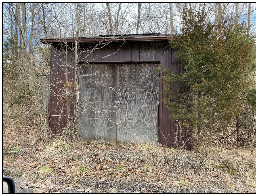
Figure 46: Old Compressor Building-Rail Car Handling
