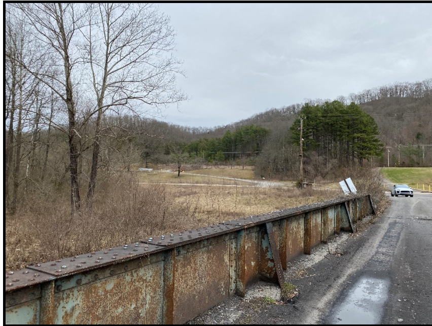
Figure 3: Northeastern Adjacent Property – (Vacant)
