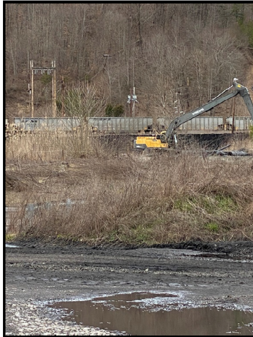
Figure 17: Pole Mounted Transformer (1 of 2)
