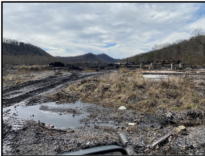
Figure 34: Property Looking West-Former Thermal Dryer Concrete Structures
