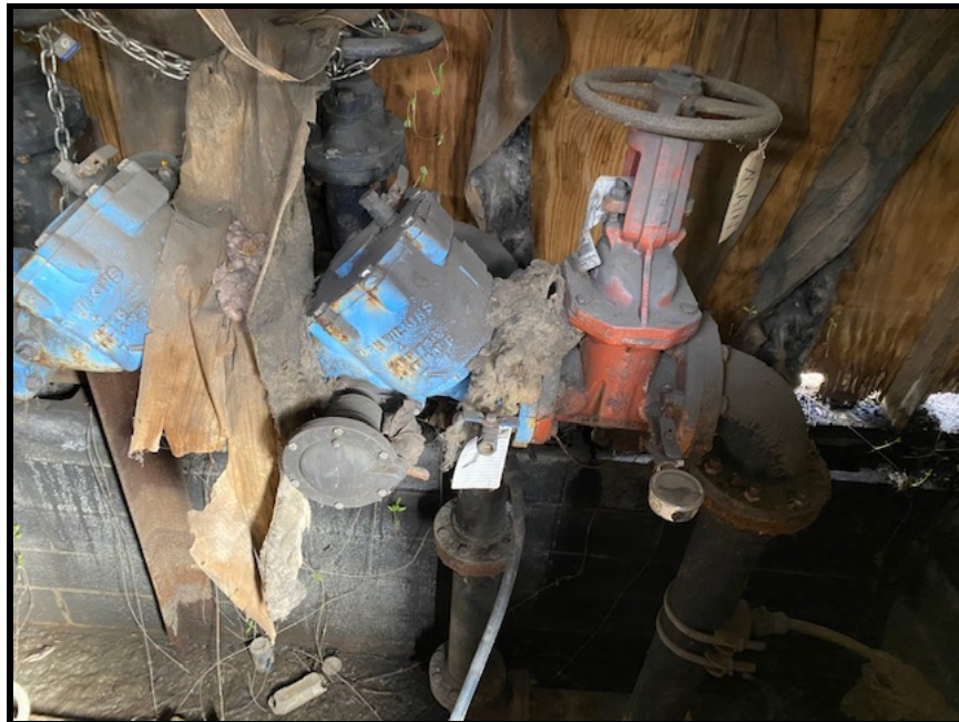
Figure 10: Water Valve Building-PSD Flow-Inside
