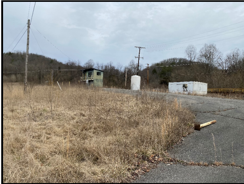
Figure 31: Old Scales - Northeast Portion of Property
