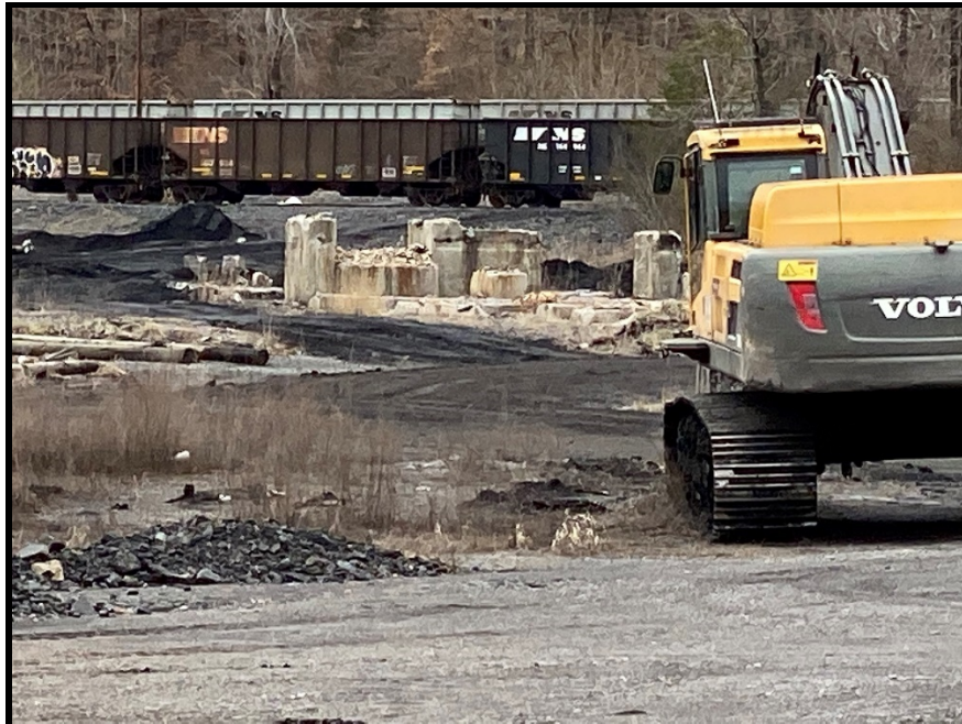
Figure 16: Western Adjacent Properties NS Railroad-Transfer Property-Concrete (Former Thermal Dryer)
