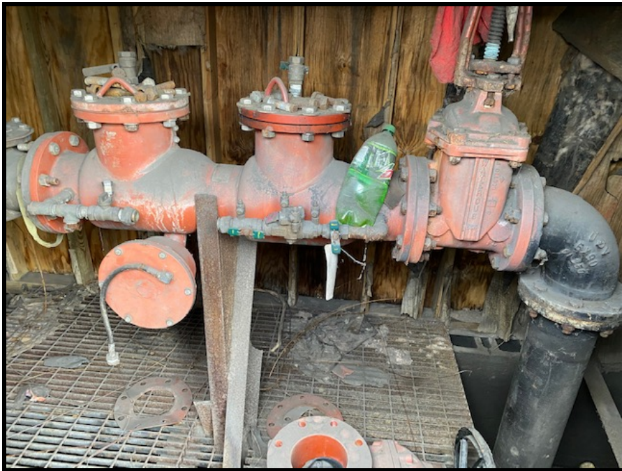
Figure 12: Water Valve Building-PSD Flow-Inside
