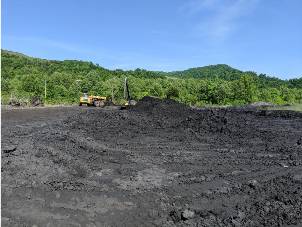
Material Excavation and Removal in Zone 1
