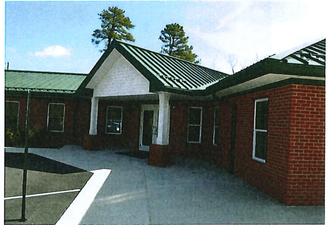
Completed New River Resource Authority Administration Building Expansion
