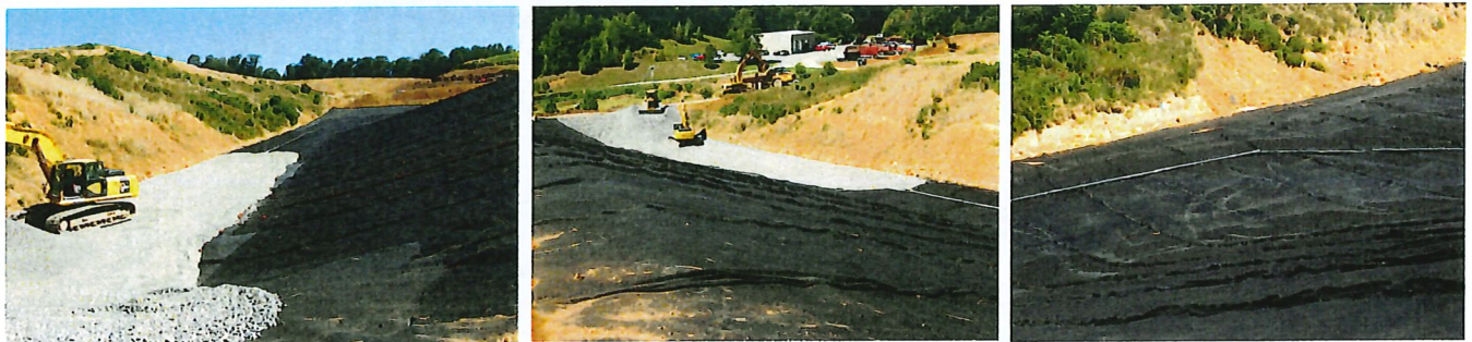
Tazewell County Landfill Expansion Phase IVA - 2007
