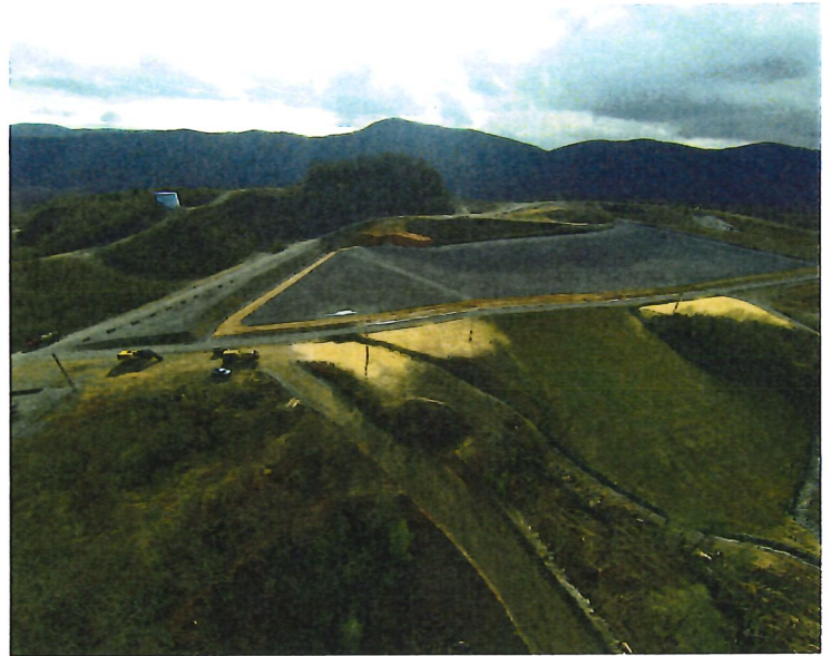
Phase IVB -Construction Complete - 2013
