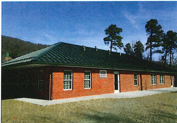
Completed New River Resource Authority Administration Building Expansion
